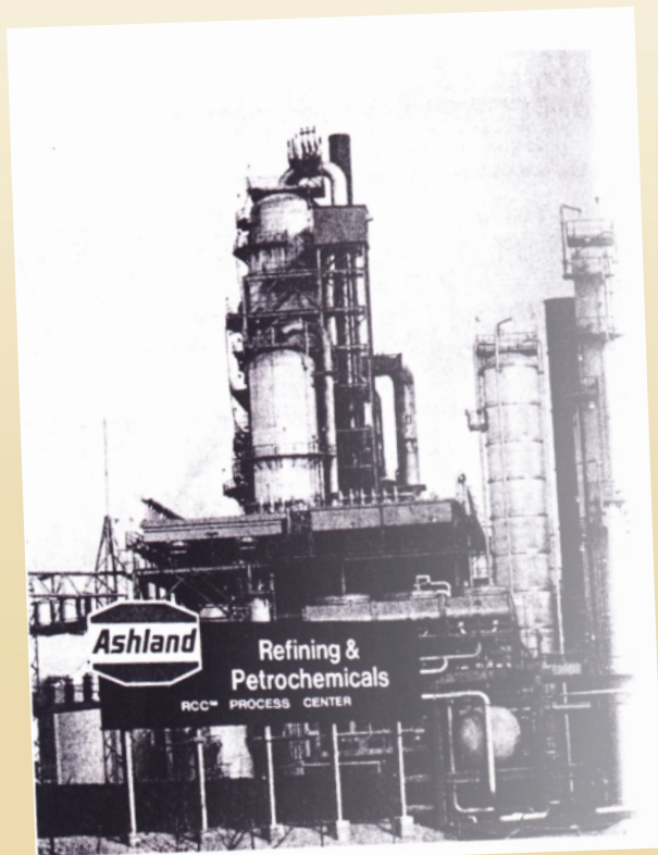
Ashland Petroleum introduces RCC (Reduced Crude Cracking) with 40,000 blb/day plant.
